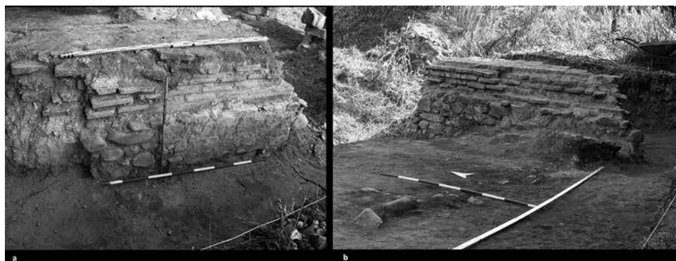
Fig. 2 Eastern wall of tower S4 from the south-east (a), from the south-west (b) (photo: S. Petković)
