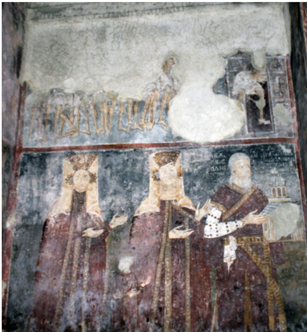
Fig. 3. White Church of Karan, northern wall of the western bay
