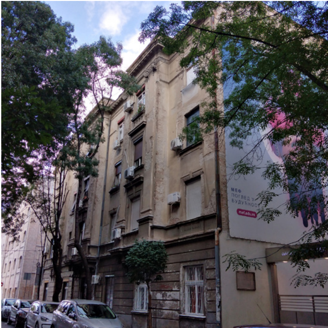
Fig. 5. Residential and commercial building for the bank officials (1921–1925), on the corner of Jevrejska and Mike Alasa streets (photo: Verica Pavićević)
