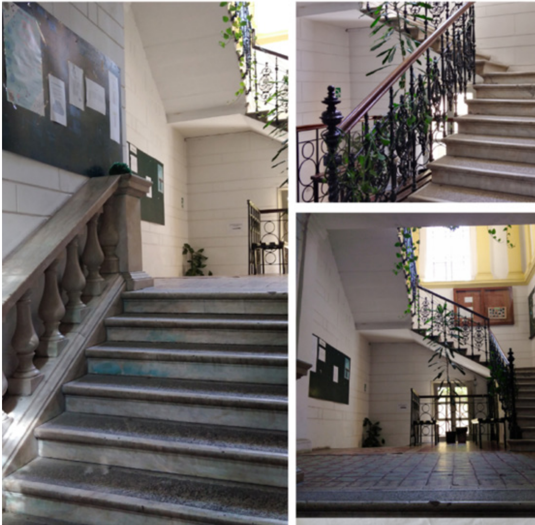
Fig. 1. Popović brothers' house entrance interior (1900), corner of Simina and Dobračina streets (photo: Verica Pavićević)
