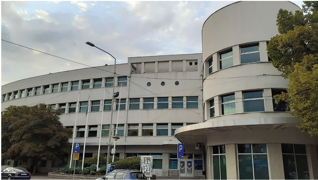
Fig. 6. A. I. Medvedev, Apprentice's Home (1939) in Nikols Pašić street 24, Niš (photo: Anđela Dukić)
