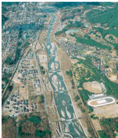
Figure 11: Japanese river with structural measure for flowing straight and rapidly Source: based on Sabo in Japan (MLIT)
