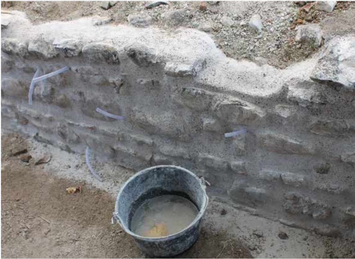
Figure 2. Restored masonry of a Roman site (Dion- Greece) (photos by the author).
