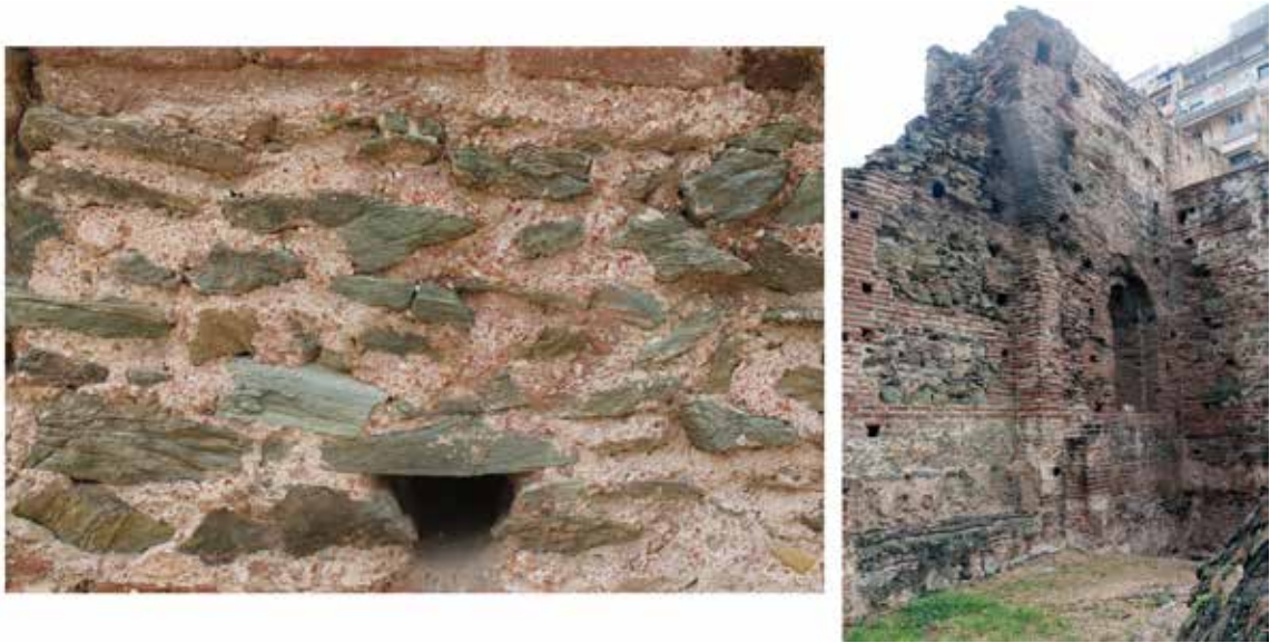
Fig. 10. (right) Cocciopesto wall joints (foundation) from the Palace of Galerius (left) in Thessaloniki (late 3 rd century-early 4 th century AD) (Dilaria in press).
