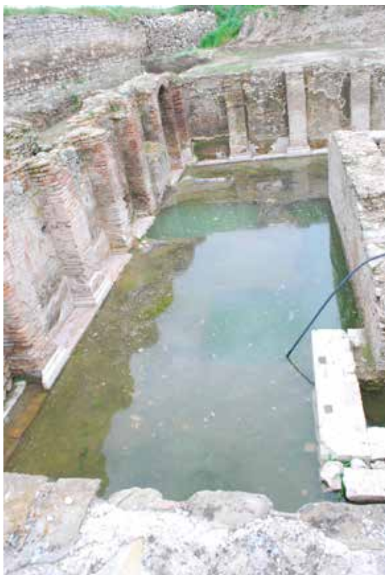
Fig. 3. Risk from flooding: rise in the level of subterranean waters and flooding in the Building with Arches, 2010 (Archive of the National Institution Stobi).
