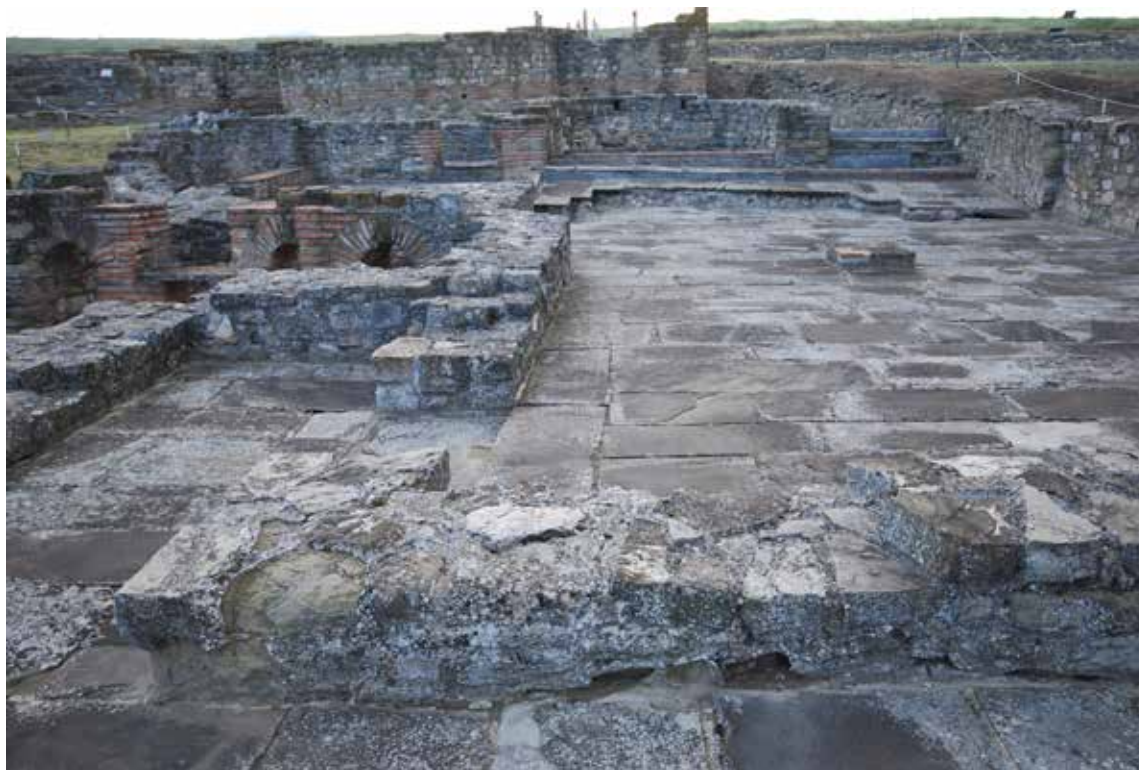
Fig. 5. Poor quality building material – soft sandstone, lichens and the use of cement-based mortar for conservation, Small Bath (Archive of the National Institution Stobi).
