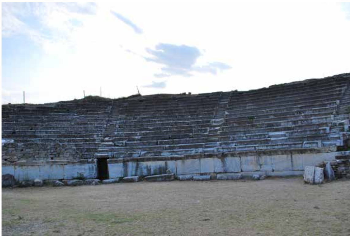
Fig. 6. Risk from air pollution: black surface on marble blocks at the Theatre, caused by exhaust gases from vehicles on the nearby motorway (Archive of the National Institution Stobi).
