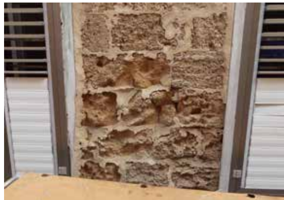
Figs. 13 and 14. Akko, Israel. Exponentially decaying calcareous sandstone after repointing with NHL pre-mixed mortar (photo by N. Copsey).
