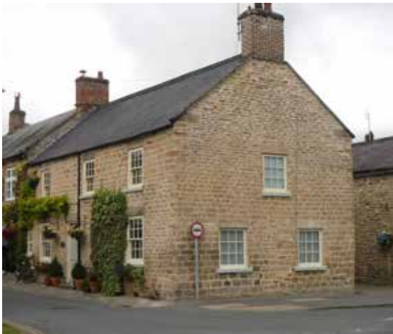
Fig. 17. Dry hot mix pointed building, "Stonehouse", Thornton-le-Dale (subject of a referenced mortar analysis by Revie) (photo by N. Copsey).
