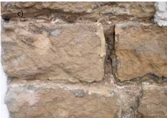
Fig. 1. The presence of residual lime lumps in earth-lime mortars from different periods and geographies: a. Masada, Israel, 2,000 years old; b. Rievaulx Abbey Cloister, North Yorkshire, 12 th century; c. bedding mortar in the wall of calcareous sandstone, Wrench Green, North Yorkshire, 19 th century (all photos by N. Copsey; c. from Copsey 2019c).
