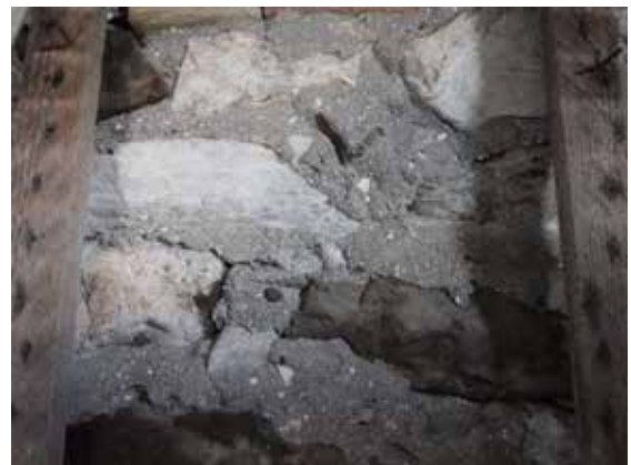
Fig. 3. Hot mixed lime mortar with basalt beach sand, Vancouver Island, British Columbia, 1864 (photo by N. Copsey).
