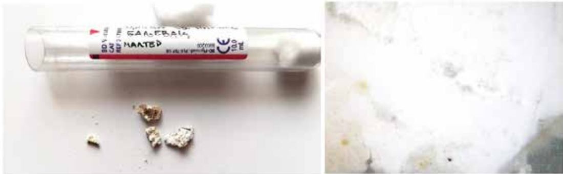
Fig. 15. Sample 1, mortar with no traces of colour. Cross-section of the sample with a magnification of ca 180x, without a painted layer on the surface (Photo by T. Tripković).
