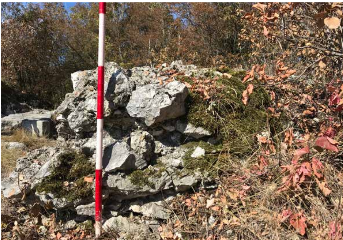
Fig. 20. Damage of the apse outer face (photo: M. Milovanović).
