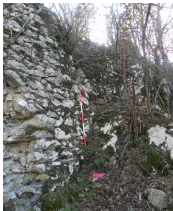
Fig. 12 The external face of the defensive wall at the central part.
