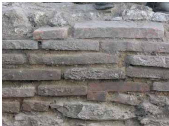
Fig. 2 Brick wall of Viminacium thermae. Photo-documentation of Institute of Archaeology Belgrade
