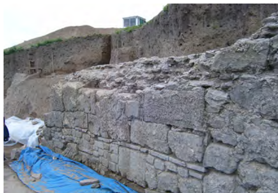
Fig. 29 Arched wall of the amphitheatre with visible bigger and smaller pieces of stone. Photo by the author.
