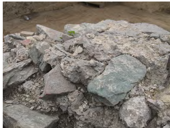
Fig. 24b Trpanac in the arched arena wall of the Viminacium amphitheatre. Photo by the author.
