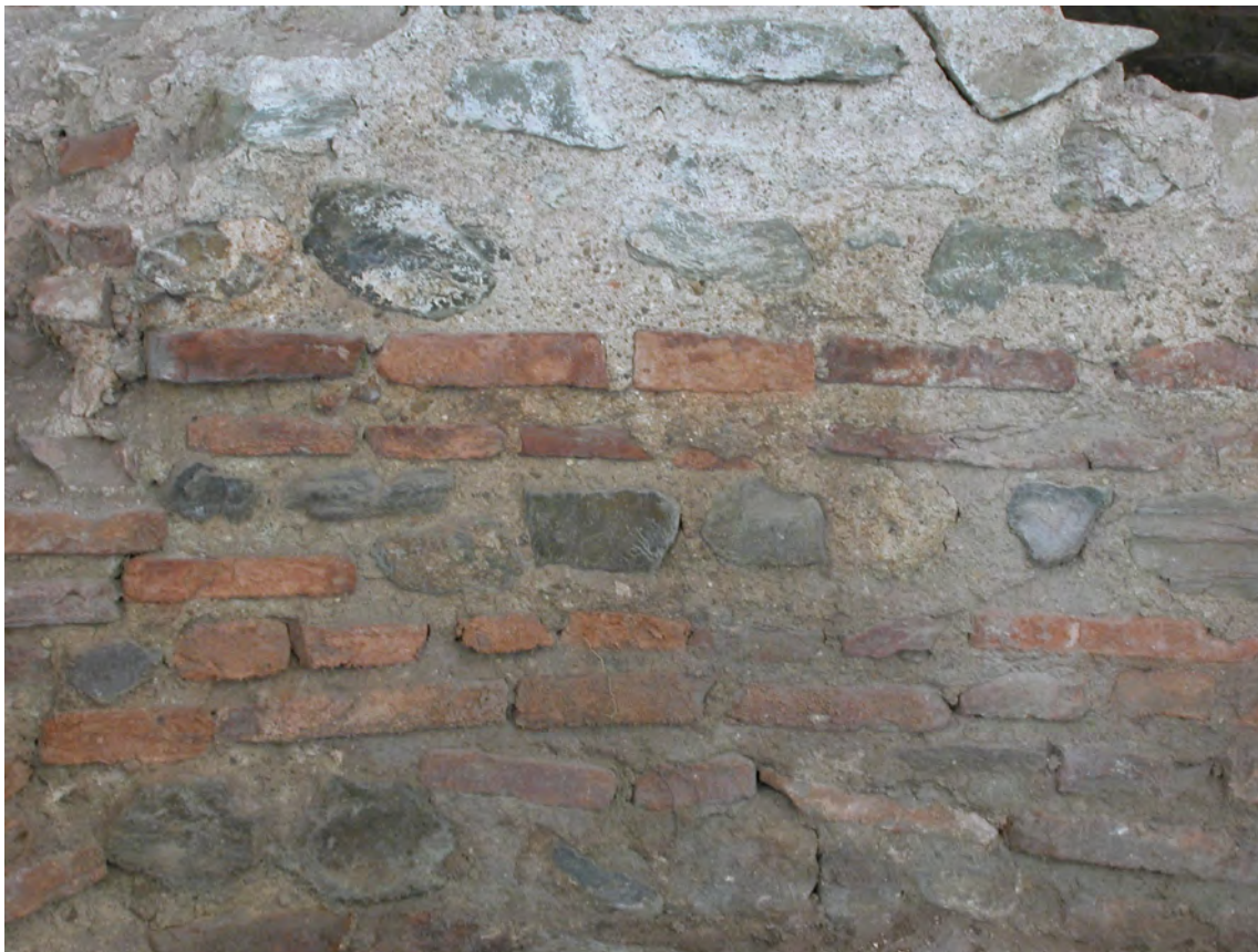
Fig. 33 Opus mixtum in the walls of Viminacium thermae. Photo documentation of the Project Viminacium, Archaeological Institute Belgrade.
