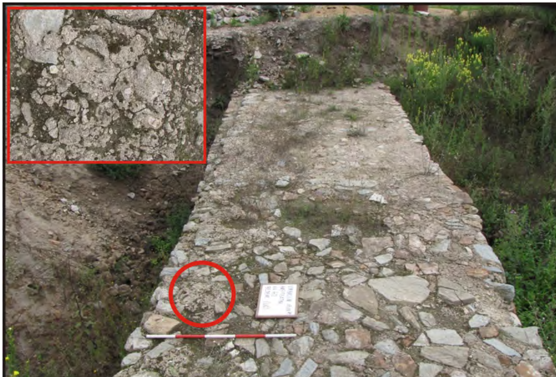
Fig. 23 Wall of the city rampart with the picture of the hard lime mortar without addition of brick. Photo documentation of the Project Viminacium, Archaeological Institute Belgrade.
