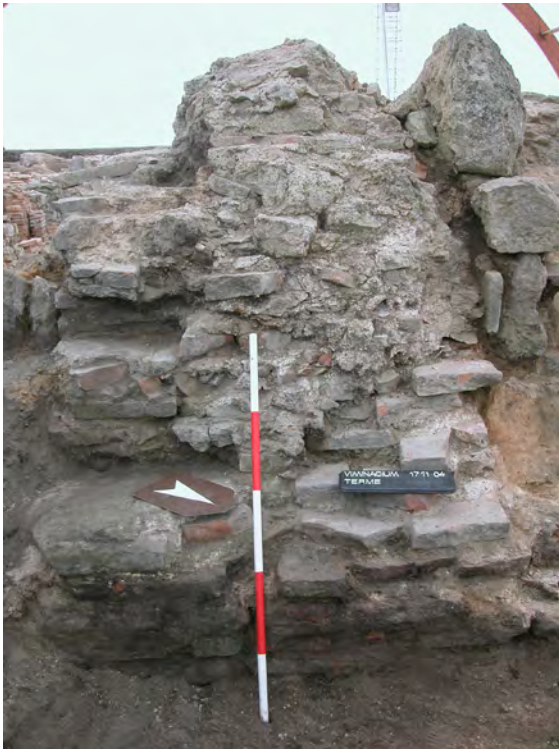
Fig. 24a Trpanac in the wall of Viminacium thermae. Photo documentation of the project Viminacium, Archaeological Institute.
