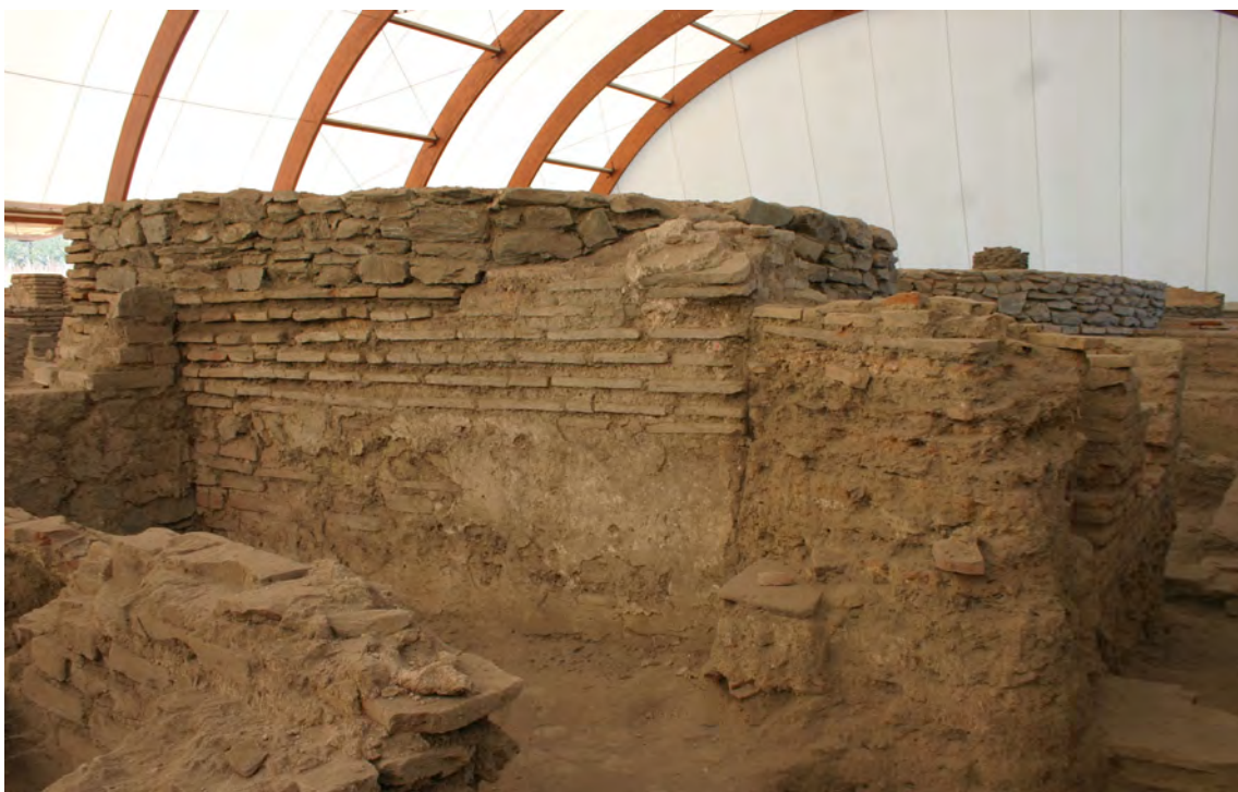
Fig. 34 Opus testaceum in the walls of Viminacium thermae. Photo documentation of the Project Viminacium, Archaeological Institute Belgrade.
