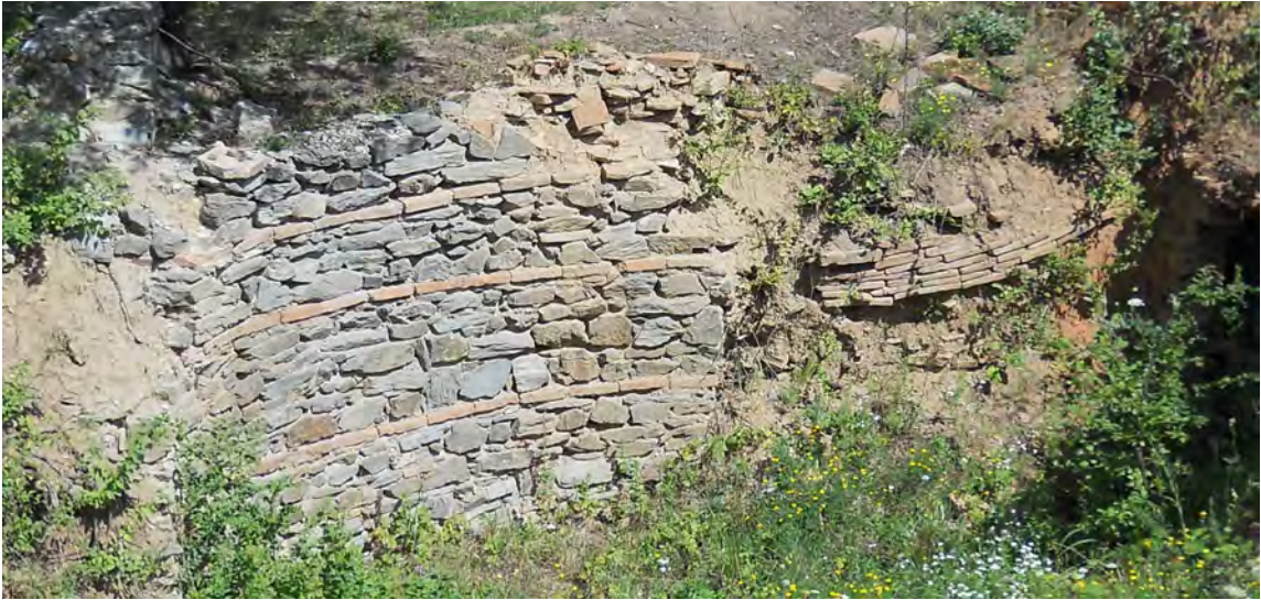
Fig. 35. Opus incertum mixtum done similarly to opus vittatum mixtum in the wall of the craftsmen's centre. Photo by the author.
