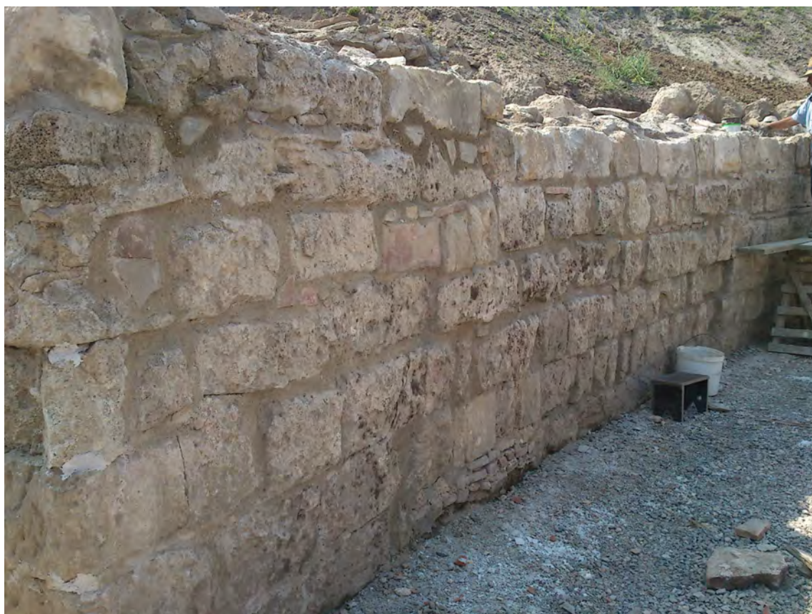
Fig. 27b Arched wall of the amphitheatre arena, detail. Photo by the author.
