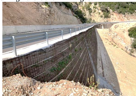
Figure 8 GRS retaining wall (Huesker).
