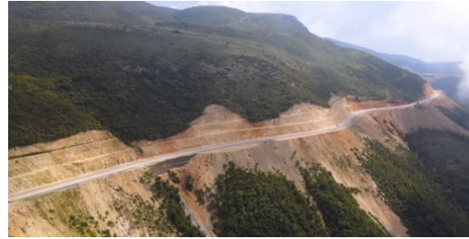
Figure 6 Cut and fill sections (TIRANA post, www.tiranapost.al).
