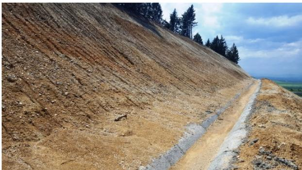
Figure 1 Soil slope with expressed erosion of the Highway Miladinovci – Shtip, R.N. Macedonia.
