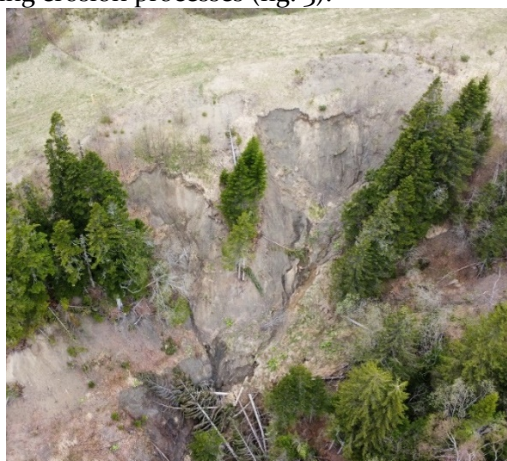
Figure 3 Landslides and erosion processes on the pipeline route.
