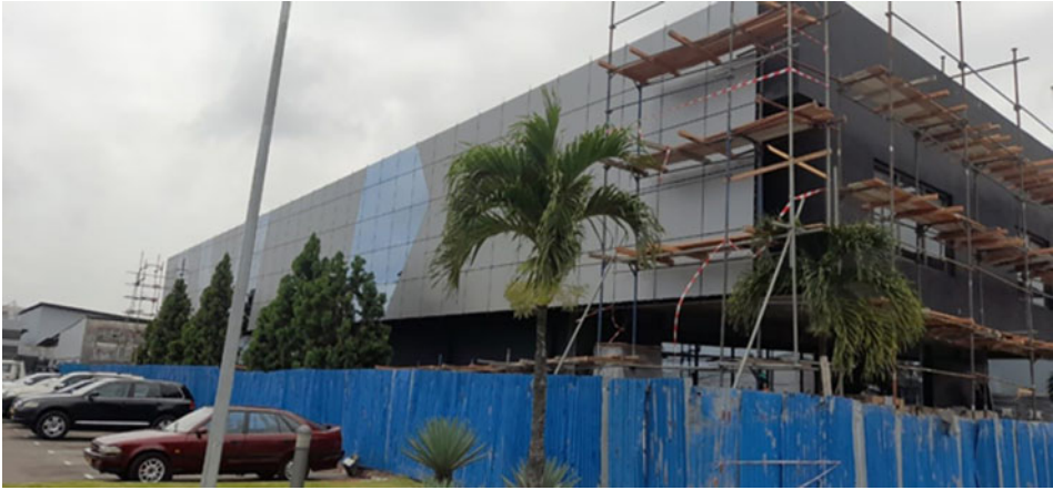
Figure 2: Central archive building during construction
