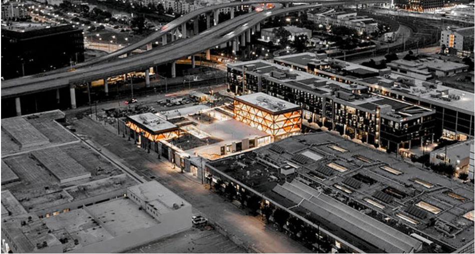
Figure 1. Exterior View and Courtyard (Photographed by the Author)
