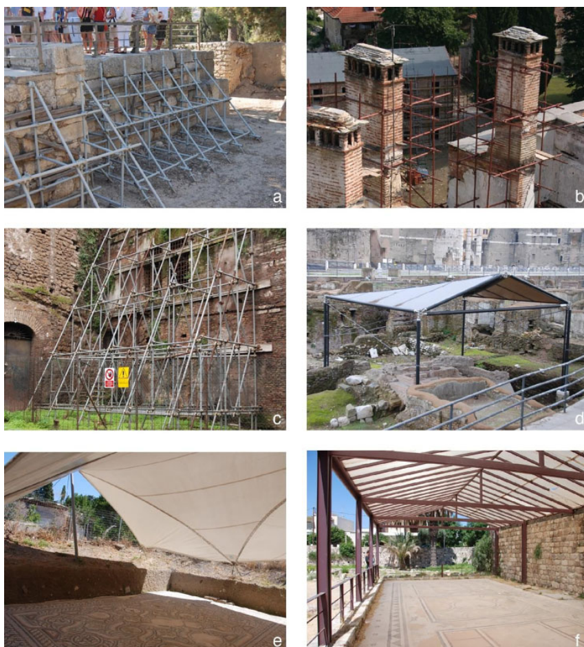
Figure 2: Temporary protective structures: a. Temporary protective structure, Knossos, Crete, b. Temporary protective structure of chimneys within the Hilandar monastery, c, d. Temporary protective structure, Forum Romano, Rome, Italy, e, f. Permanent protective structure, the town of Kos, Kos, Greece. Source: Authors.
