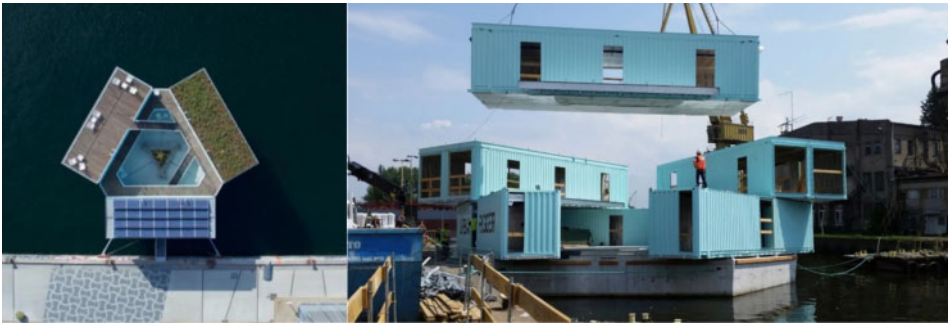
Figure 3: Top-down view of modular Urban Rigger unit with solar and green roof, Construction process of Urban Rigger using upcycled containers - https://big.dk/projects/urban-rigger-3021
