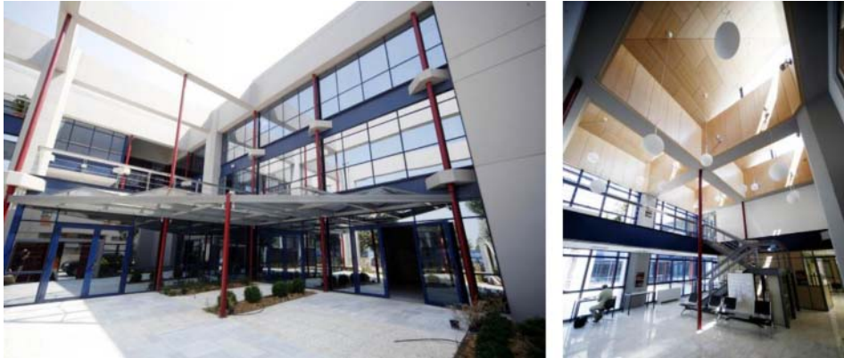
Figure 1: External and internal (1 st floor) view of the building under examination.
