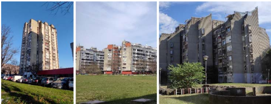
Figure 1: Examples of residential buildings in Central Zone of New Belgrade
