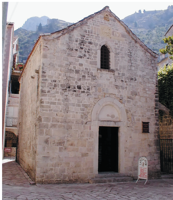
Fig. 4 Church of St. Michael – after the works
