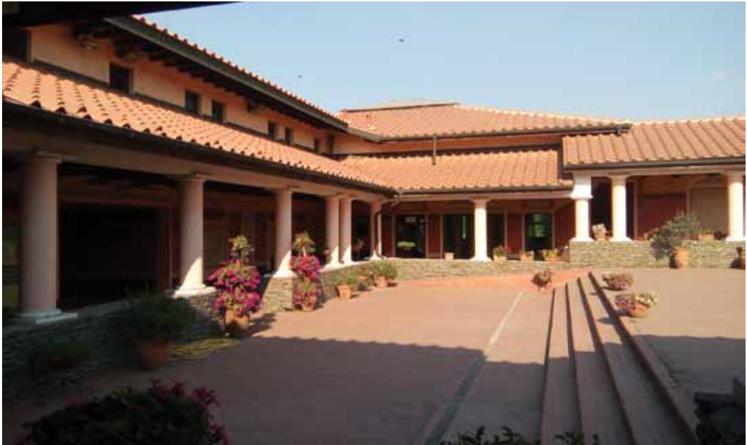
Fig. 2. Access ramp in the Domus Scientarium Viminacium atrium, Viminacium Archaeological Park (source: Documentation of the Institute of Archaeology in Belgrade)
